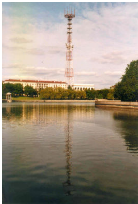
Right behind the Belarus Radio and reflected in the Svislach river, is the telecommunication tower. From here the signals are carried by microwave to SW transmitter site at Kalodiziscy, 15 km. East of Minsk.
