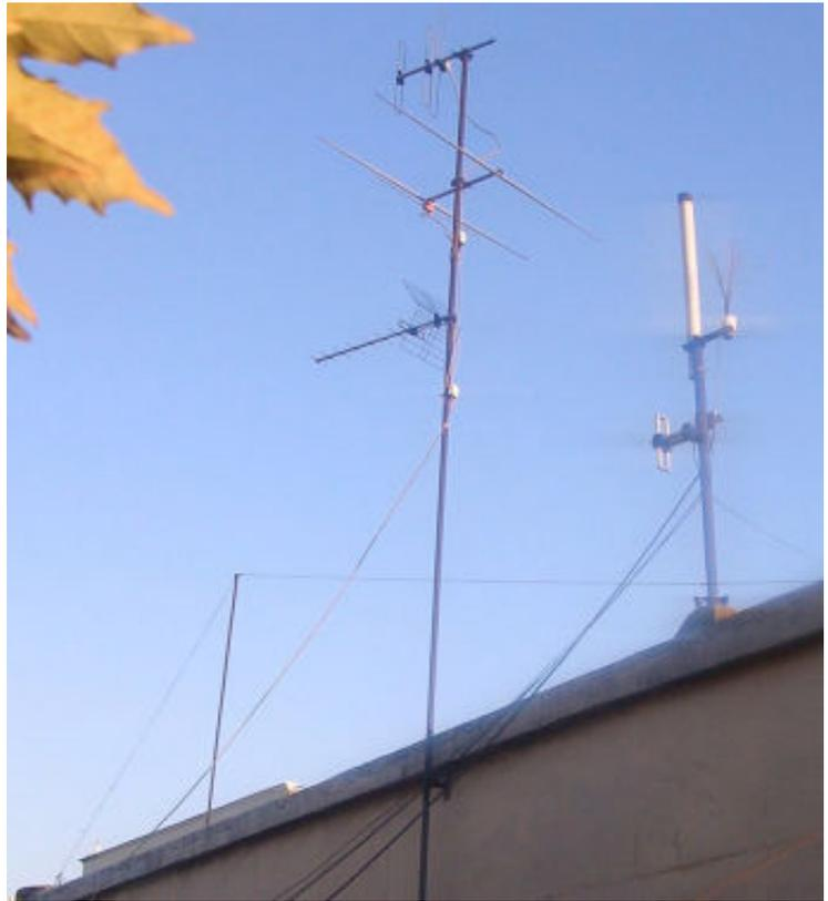
There are 6 antennas installed on the roof of Radio Tirana, and the main one has the form of the Russian letter G, which is what I call an 'L-antenna'. Others also cover VHF and UHF, besides MW and HF. The photo, taken on November 26, 2004 shows the antennas.
